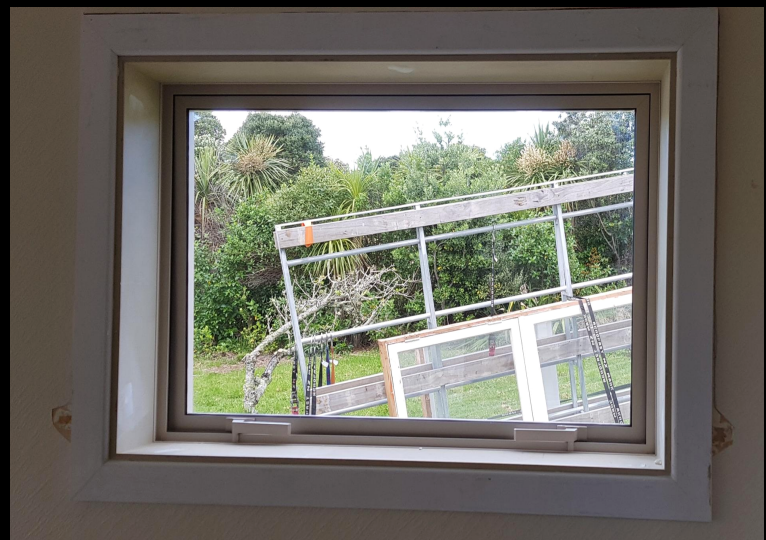
Cut & Fit internal architraves.
