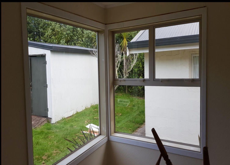
Cut & Fit internal architraves.
